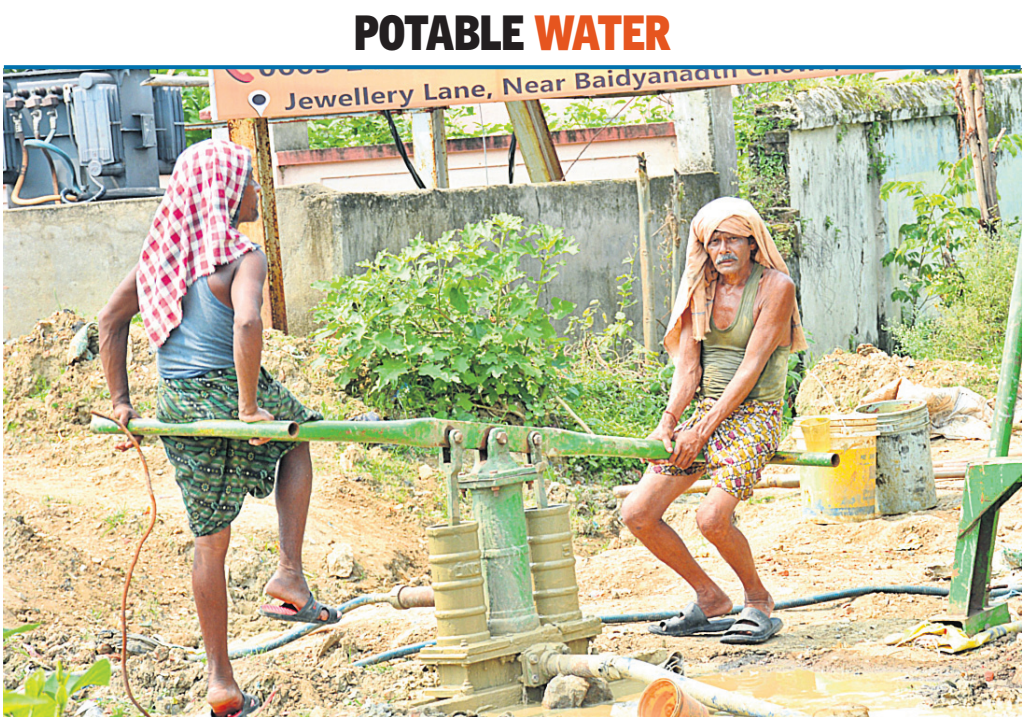
Workers sinking a tube well at Baidyanath Chhak in Sambalpur
