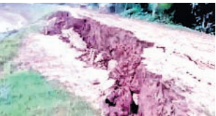
A part of the river embankment at Rameswarpur under Dhamnagar block caves into Genguti river
