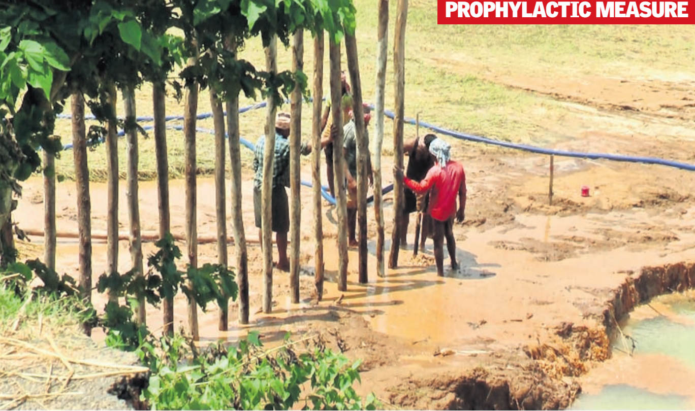
A breach on an embankment of Kelua river in Dharmashala area of Jajpur is being repaired
