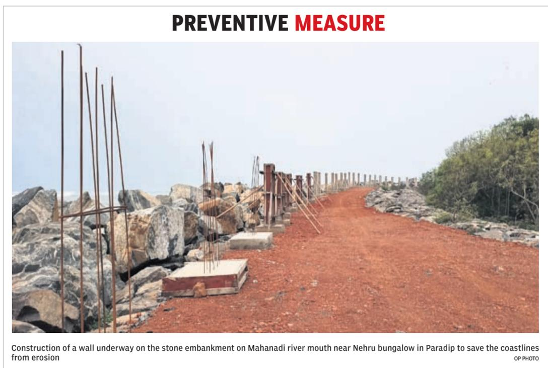
Construction of a wall underway on the stone embankment on Mahanadi river mouth near Nehru bungalow in Paradip to save the coastlines from erosion
