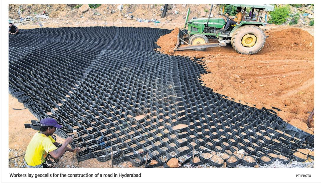
Workers lay geocells for the construction of a road in Hyderabad
